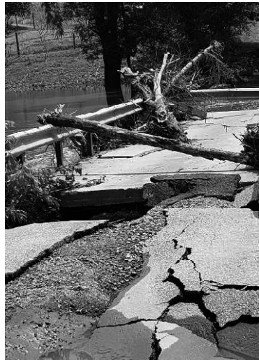
SASS Ave Bridge
